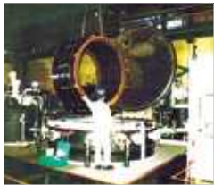
Impregnation of core and coil assemblies
